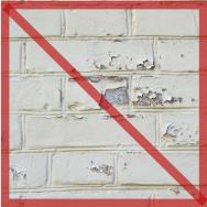
Mineral paint will never peel from brick. Here, ordinary acrylic latex paint is peeling due to moisture escaping from the masonry surface.
