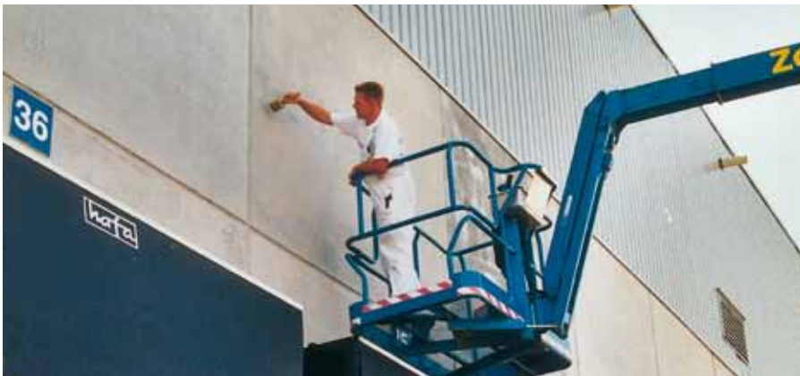
KEIM service technician at work
