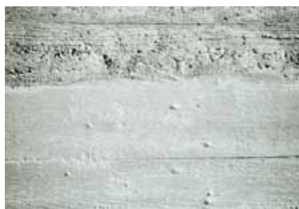
Blowhole grouts, brushed on, coarse board formwork texture retained
