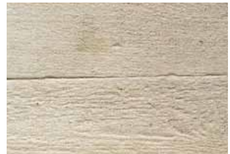
Scratch filler, applied with sponge float or hard rubber float Board formwork texture retained
