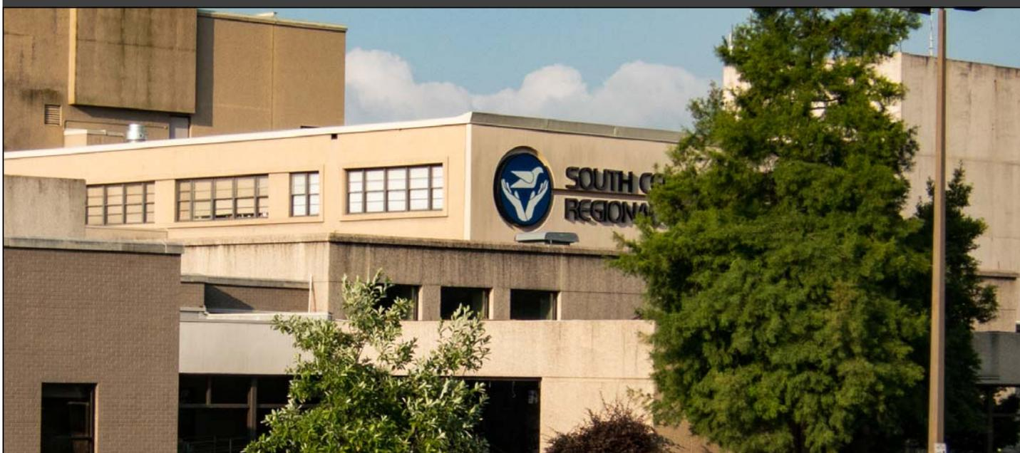
The panelized construction does not match in either color or texture with the brick façade. To hide the appearance between these surfaces and present a professional appearance, painting was the only answer. It was first painted about 1989 when the hospital converted from Jones County Hospital to South Central Regional Medical Center. The second repainting cycle was in 1999. Each time the acrylic polymer paint was noticeably faded, chalking, and surfaces discolored after just five years.
